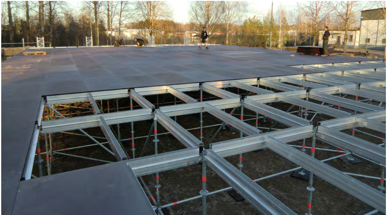
Photo: Prolyte Sales, Space Roof training Starlight
